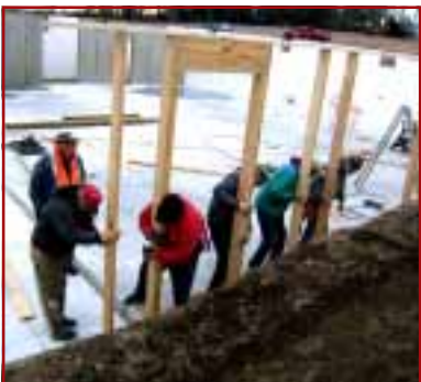
Dec. 27: Framing north wall.
