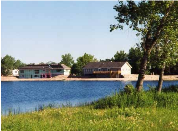
High-density building development on a sandpit.
